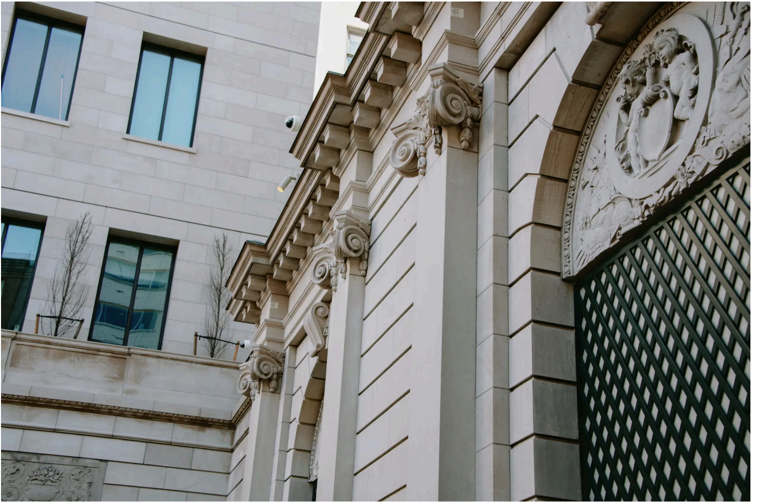
The new limestone-clad addition, left, overlooking the garden, steps back for a row of hornbeams.
